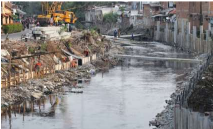
Figure 2. Condition of the Ciliwung Riverbank management in RW 08, Kampung Melayu Subdistrict through the construction of retaining walls as an effort to control flooding. Source: https://megapolitan.kompas.com
